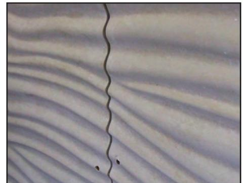
4. Install your first panel at the bottom corner of the wall. Double check to make sure your panel is level and parallel to the wall. Mastic or Liquid Nails (behind the panel) can be utilized to hold the piece in place. Start screwing in the panel, working your way from the top to the bottom. Continually check the alignment of the panel while placing screws to ensure it has not been tweaked. (Note: Carefully tighten the screws down, over tightening may cause the panel to crack)
