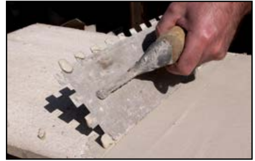
Apply a thin polymer-modified thinset bond coat to the back of the stone.
