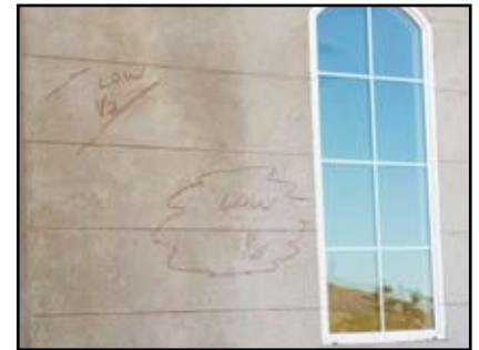
Mark all the low areas and use thinset to level them out to the proper height before installing Classic Series tiles.
