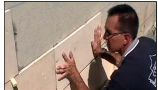
Work the stone into the wall using a left-to-right motion until the mortar squeezes from the perimeter of the tile and full-coverage adhesion is achieved.
