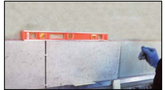
Using a propped up rigid aluminum channel can help you support and level out the first row of tiles during installation.
