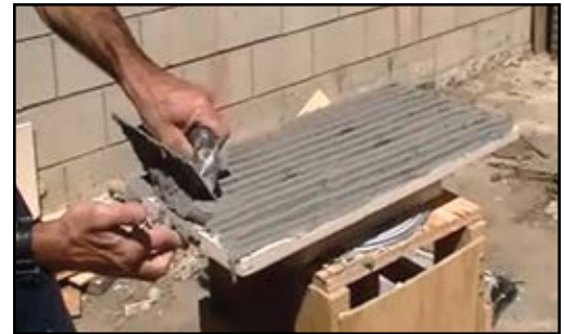
Use a 1/2" notched trowel to apply non-sag polymer-modified thinset bonding mortar to the back of the stone.
