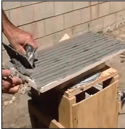
Use a 1/2" notched trowel to apply non-sag polymer-modified thinset bonding mortar to the back of the stone.
