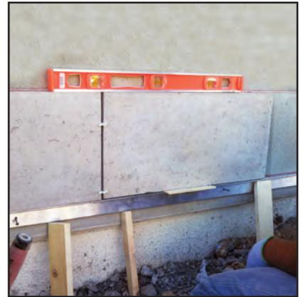
Using a propped up rigid aluminum channel can help you support and level out the first row of tiles during installation.
