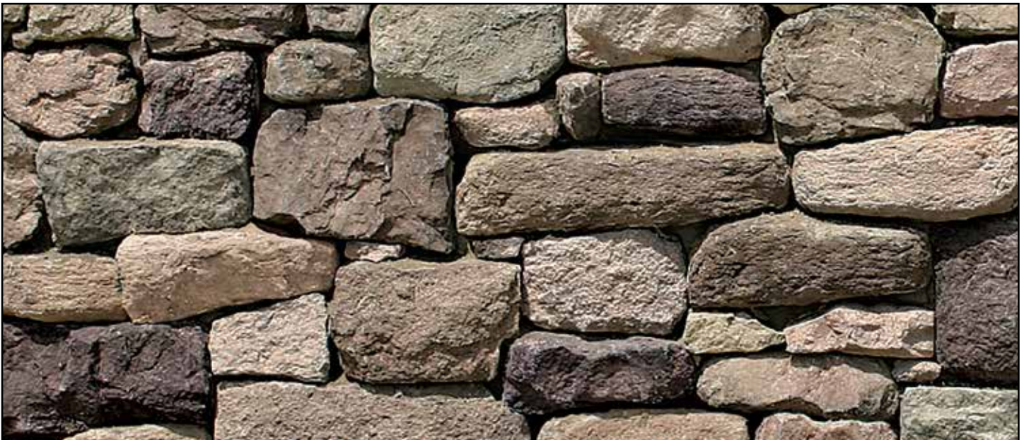
Drystack to ½" Grout Joint
